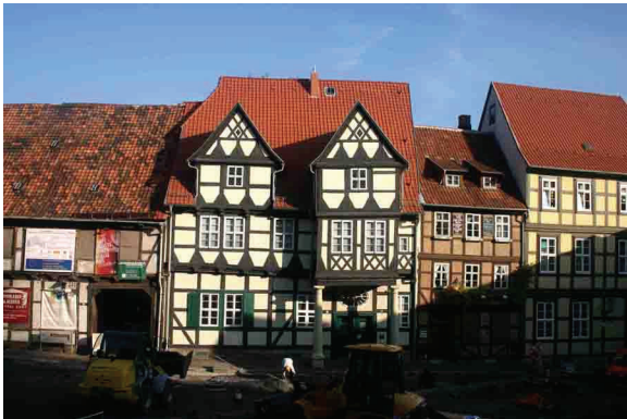
Buildings so close-packed they hold each other up
