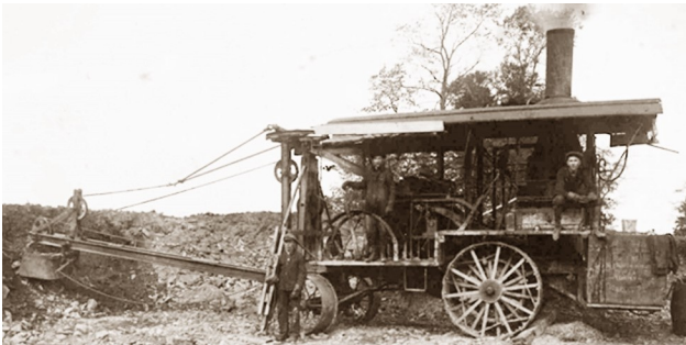
Roy Knox operating a Keoring Excavator in the Rintoul Quarry, ca. 1921 (MGR093-001)
