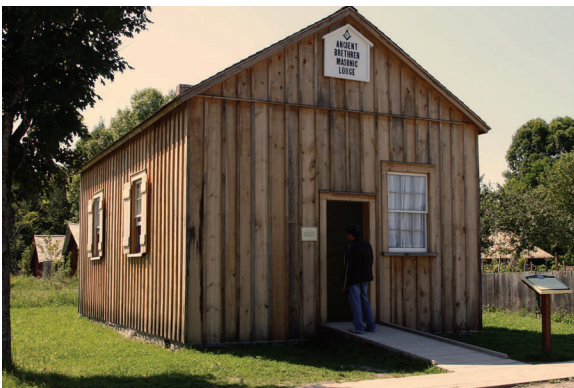
Restored hall at Upper Canada Village
