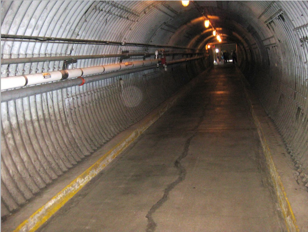
The tunnel entrance to the bunker proper
