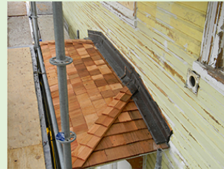
New shingles on front door canopy
