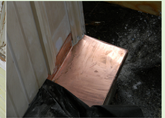
New copper flashing at ground level
