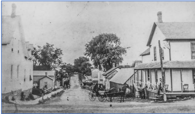
View down Burritts Ave./Grenville St. from Donnelly Drive
