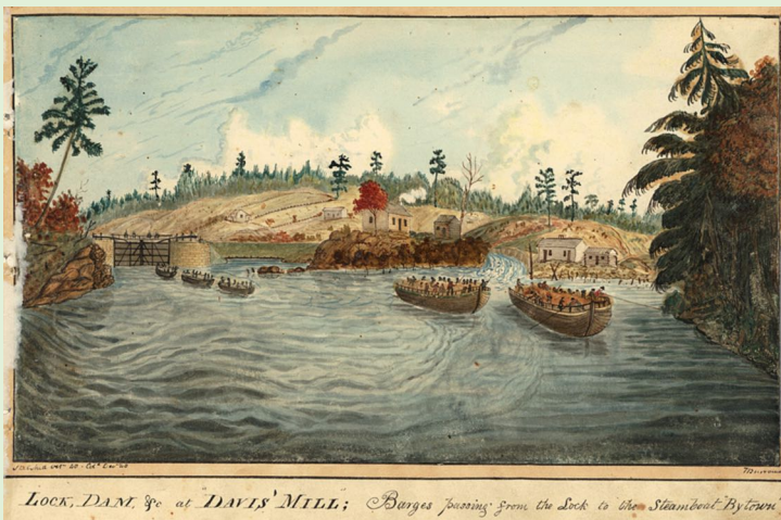
LOCK, DAM, &c. at DAVIS' MILL; Barges passing from the Lock to the Steamboat 'Bytown'. Sketched Oct. 40. Col.d Dec. '40, 1840; Thomas Burrowes fonds; Archives of Ontario.
