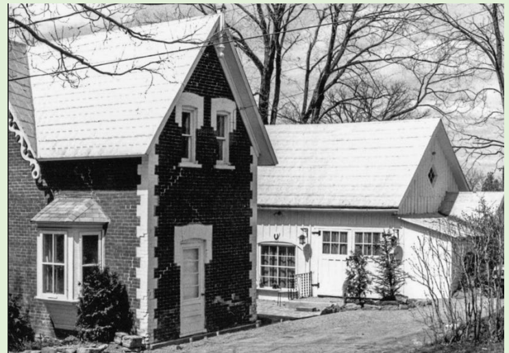
View from Currier St. showing carriage shed (c.1950s)
