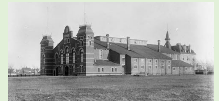
Cartier Square Drill Hall
